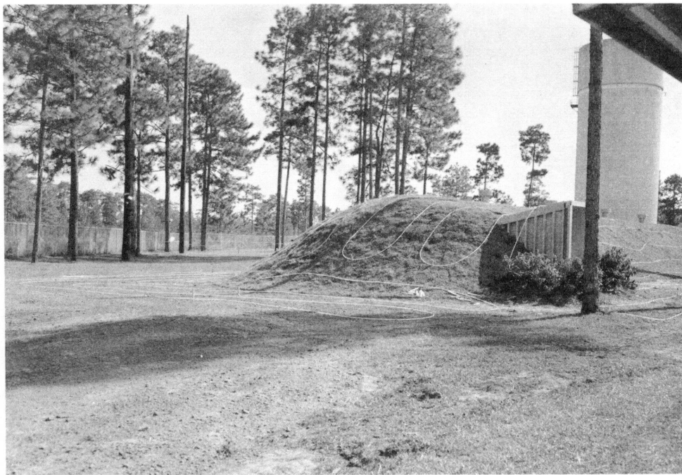
Fig. 2.14— Tubing layout at shelter.
